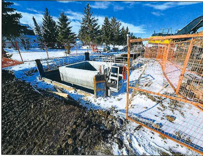
SPS - Precast installation
