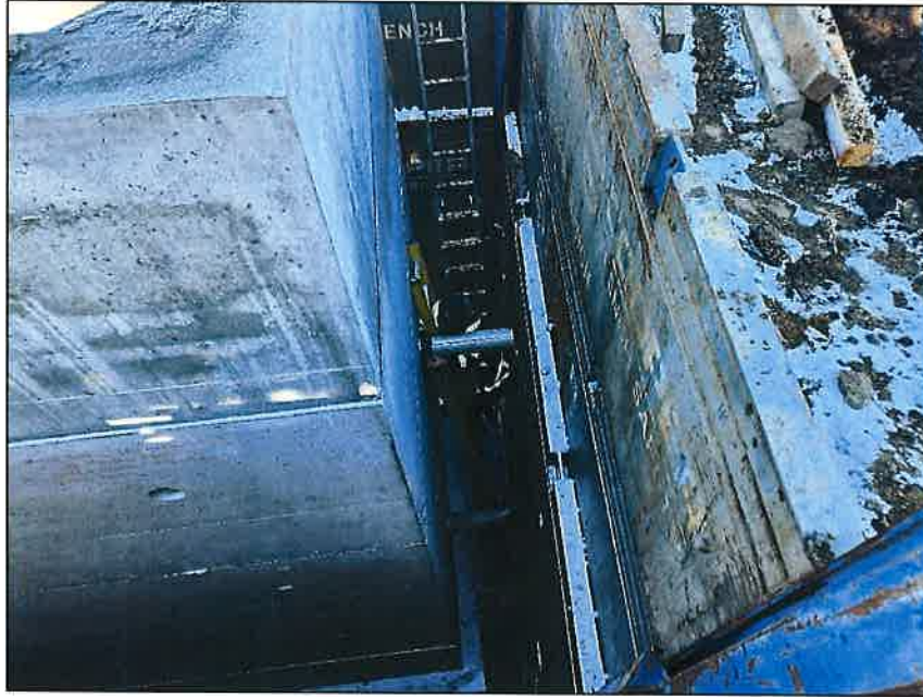
SPS - Precast installation
