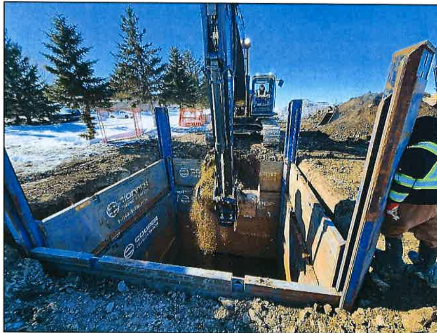
Sewage pumping station excavation
