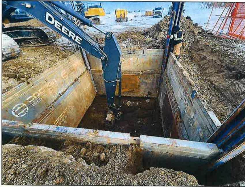
Sewage pumping station excavation
