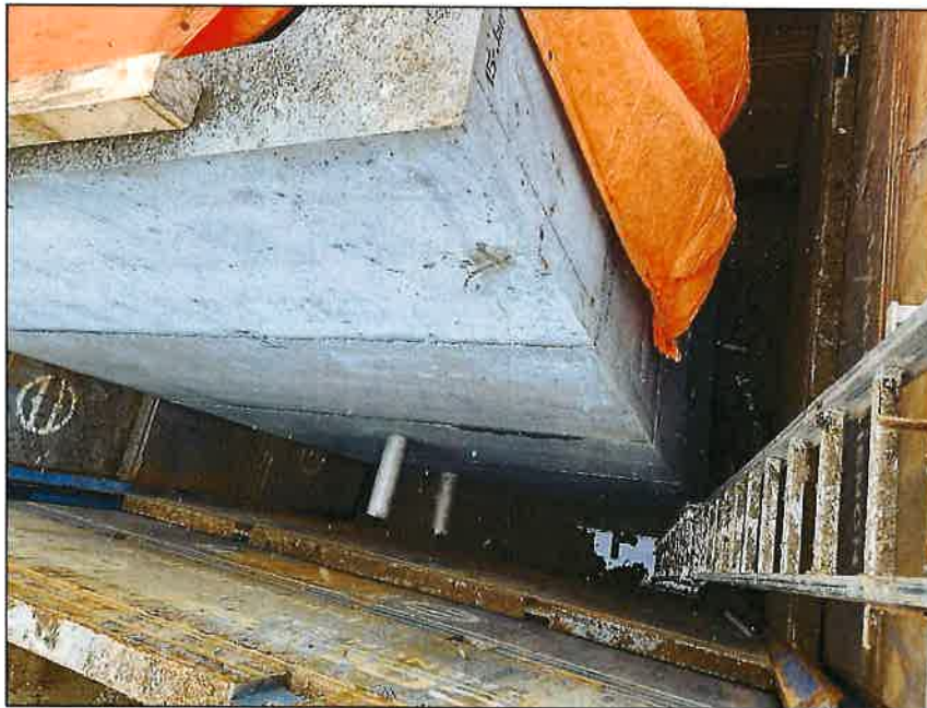
SPS - Precast installation
