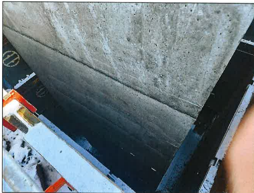
SPS - Precast installation
