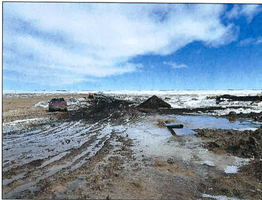
Sewage force main installation – tie-ins
