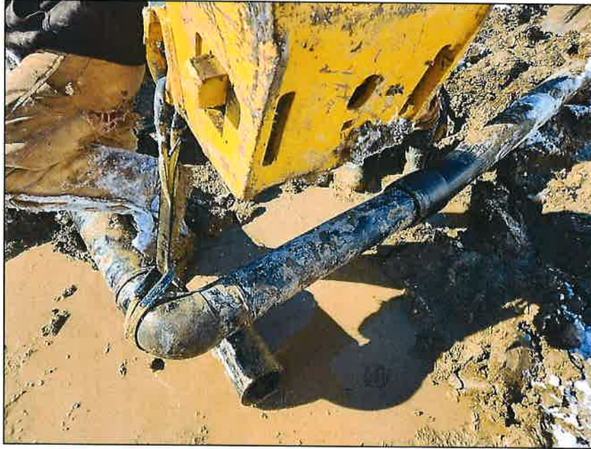
Sewage force main installation – tie-ins
