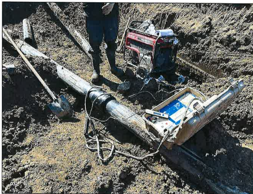
Sewage force main installation – tie-ins
